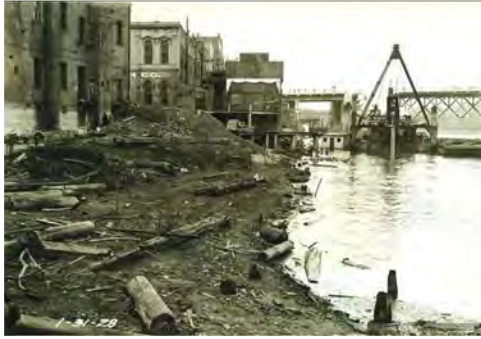
1928- Portland's West Side Waterfront Construction
