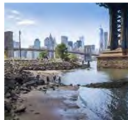
REMOVED SEA WALL REPLACED WITH FLOOD-TOLERANT STONE RIP-RAP SHORELINE
