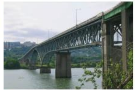
9 Ross Island Bridge
